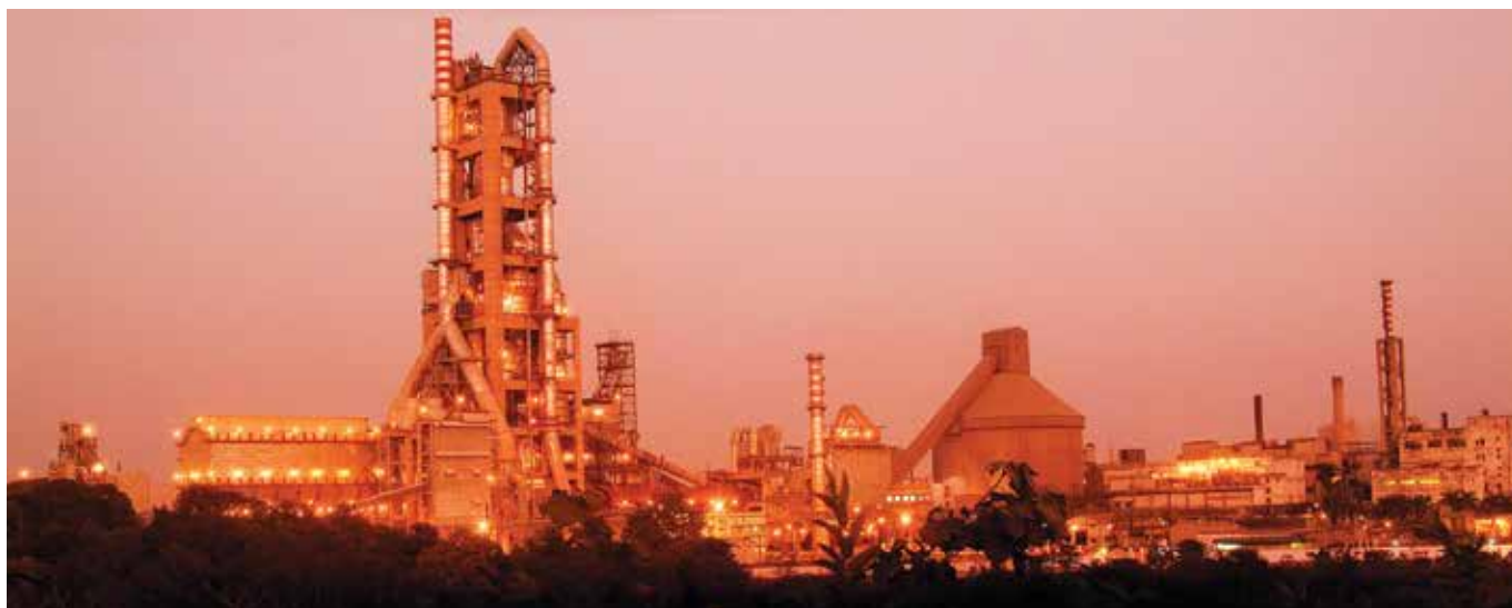
ACC Wadi Cement Plant
