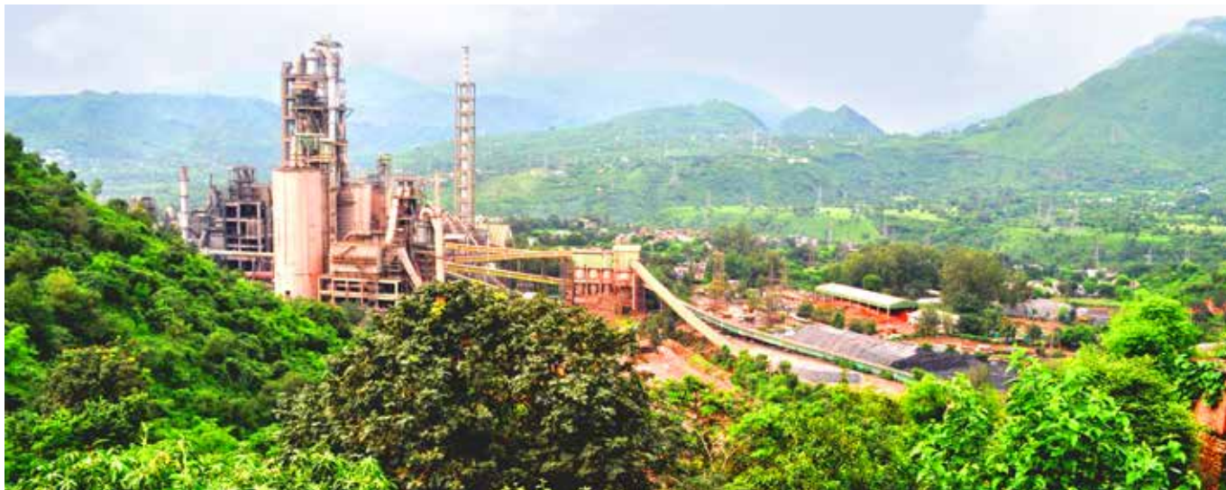
ACC Gagal Cement Plant
