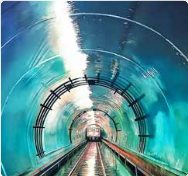
Kolkata's Underwater East West Metro Tunnel
