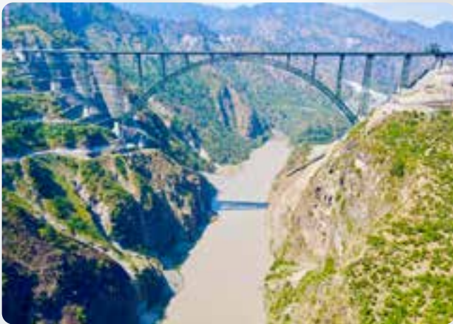
Chenab Railway Arch Bridge
