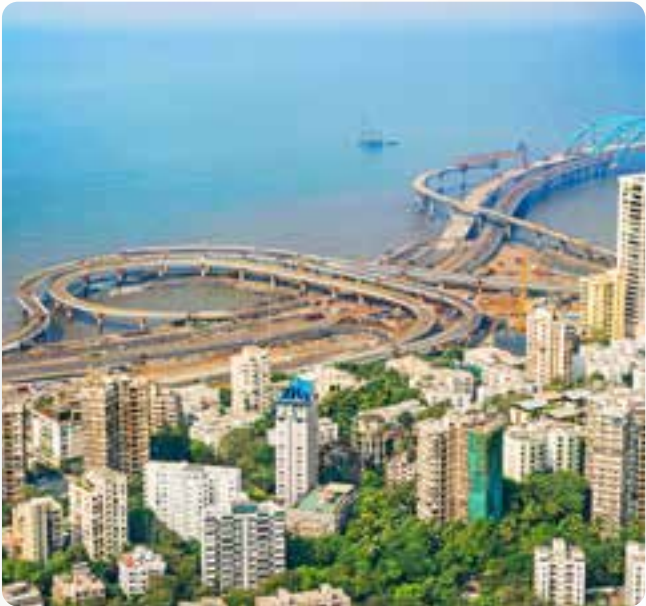
Mumbai Coastal Road Project (MCRP)
