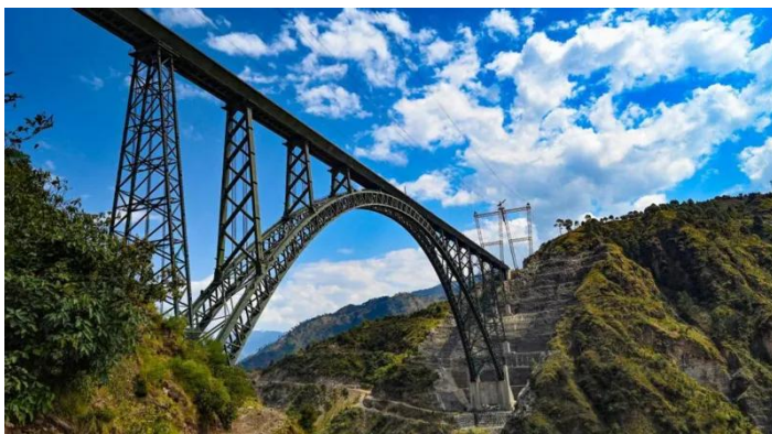
Chenab River Arch Bridge
