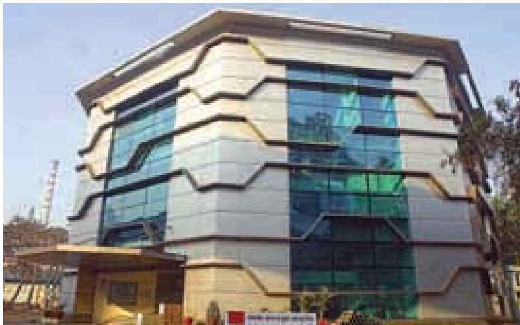
The Central Control Room Building at ACC Chanda, one of our green buildings and the first such in an industrial environment
