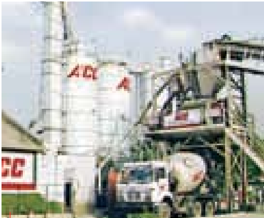
ACC Ready Mixed Concrete Plant today
