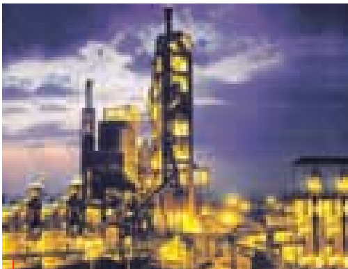
ACC Wadi Plant - 2.6 MTPA
