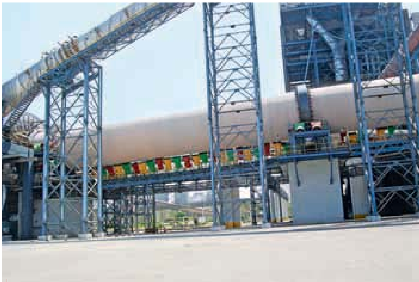
World's largest kiln at ACC Wadi, Karnataka
