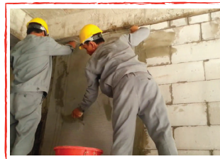
• AAC Block plastering work
