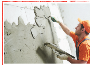
• Internal plastering of walls & ceilings
