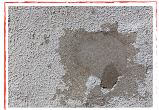
• Other general purpose repair & patch work
