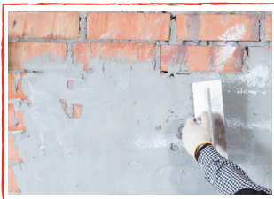
• External plastering of walls
