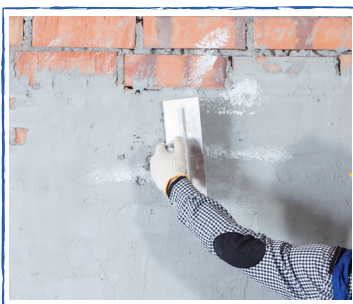
External plastering of walls
