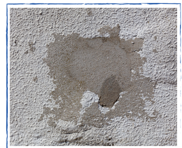
Other general purpose repair & patch work
