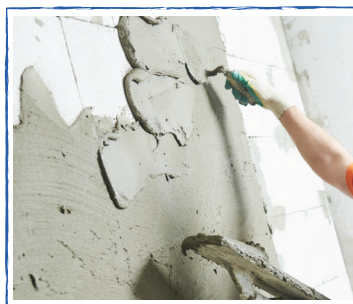
Internal plastering of walls & ceilings
