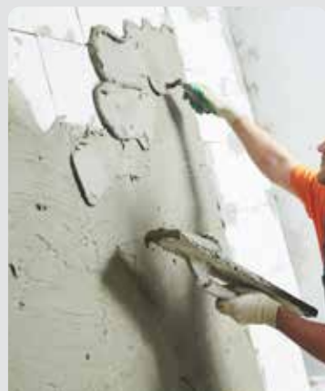
Internal plastering of walls & ceilings
