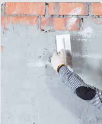
External plastering of walls
