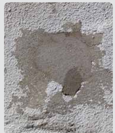
Other general purpose repair & patch work
